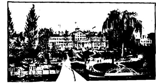
The La Tourette House in 1860 was originally a chateau built by the DuPont family in the 18th century. Sold in 1806, the mansion was converted into a hotel. For over a century, the sumptuous rooms of the hostelry made it a favorite with New York's society leaders.
